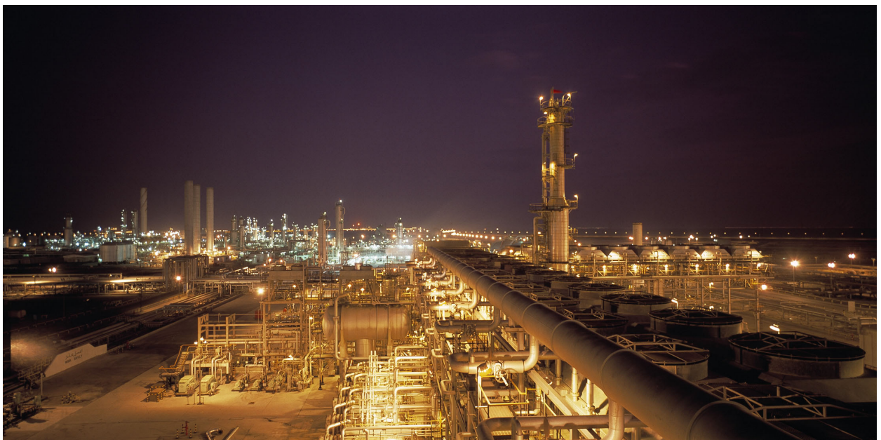
Ras Tanura Oil Refinery (Used with permission from Saudi Aramco World/PADIA)
